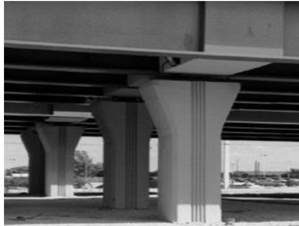
Fig. (1.15): Pier foundations.
